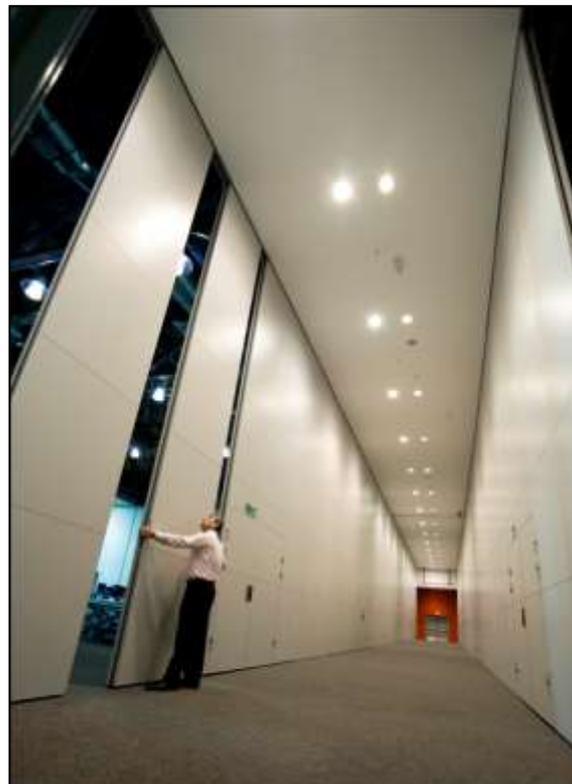
Figure 1 An example of an installed AMPW
